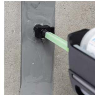
3. Insert mixer nozzle in the packer inlet spigot. Hold firmly in position and press trigger to inject.
